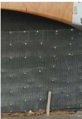
Fig.1A - Attaching Lath
