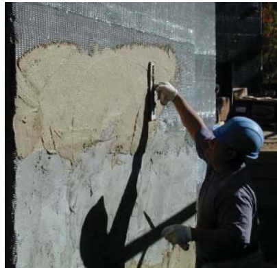
Fig. 1B - Applying scratch coat of mortar
